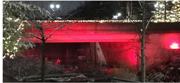
Newmarket Fred Lundy Bridge lit up red to support Red for Change, November 2023
